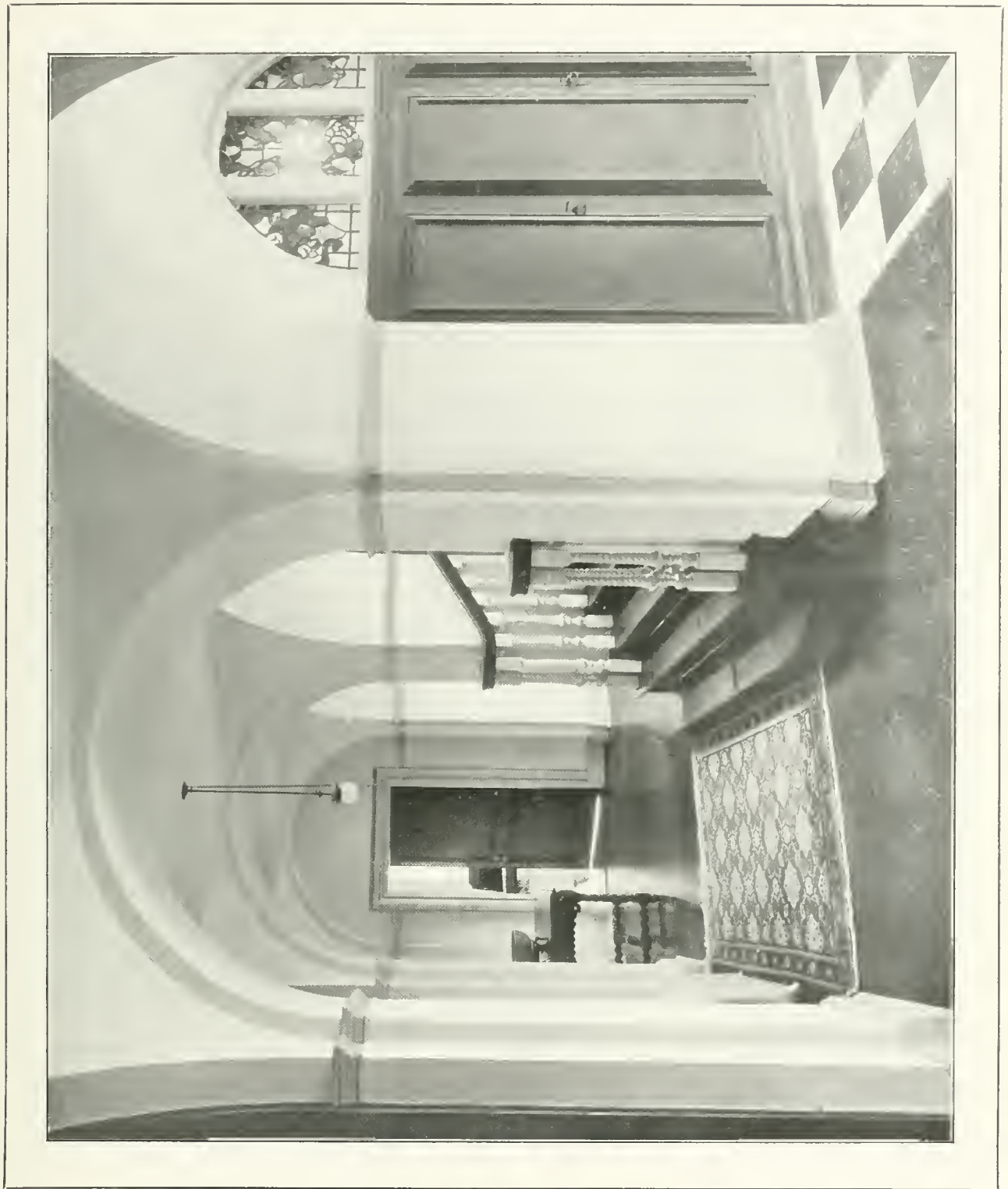
The entrance hall and vaulted corridor are simply finished in white, the latter being paved with dark-red hexagonal tiles, and the entrance hall has a floor of black and white marble squares. The hall has walls panelled with oak.
